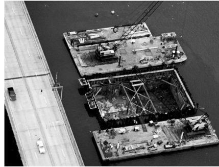
Bridge Pier Cofferdam Brunswick, GA
