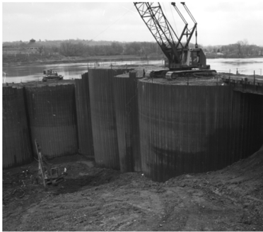
Water Intake Cofferdam Kenton County, KY
