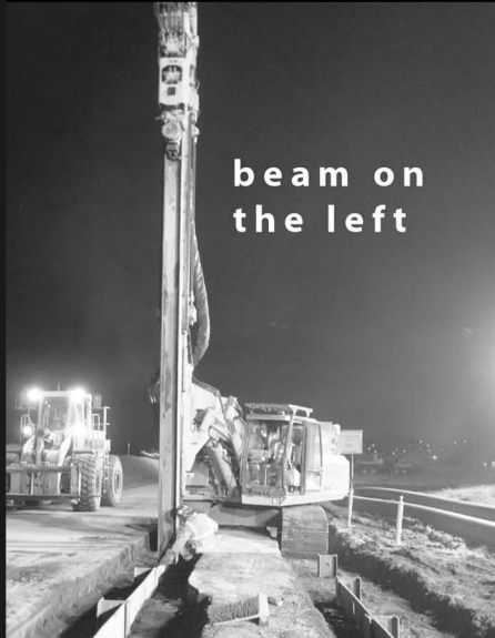
Drive sheet pile on both sides, track forward
