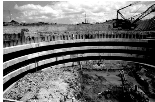
Circular Cofferdam Around Collapsed Rectangular Cofferdam Mayaguez, Puerto Rico
