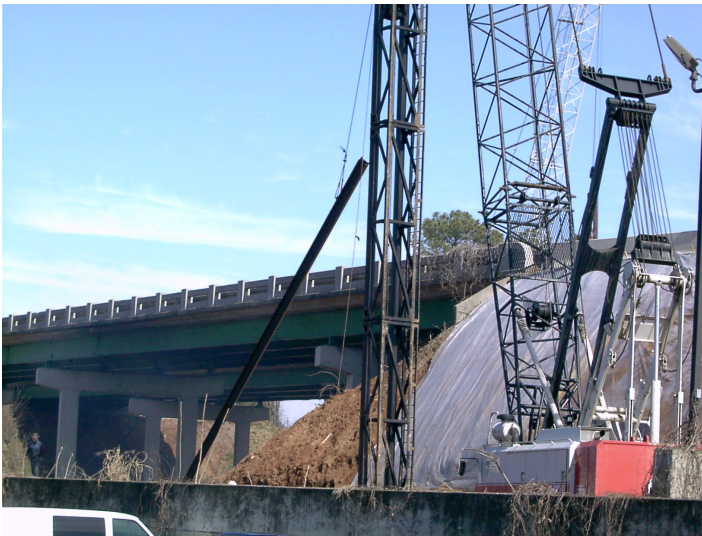
Figure 5-38 Single-Point Pickup of an H-pile
