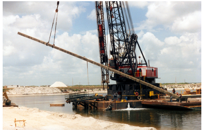
Figure 5-48 Single Point Pick-up of Concrete Pile
