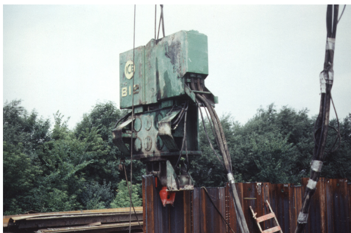
Figure 5-85 Vibratory Hammer Driving Sheet Pile
