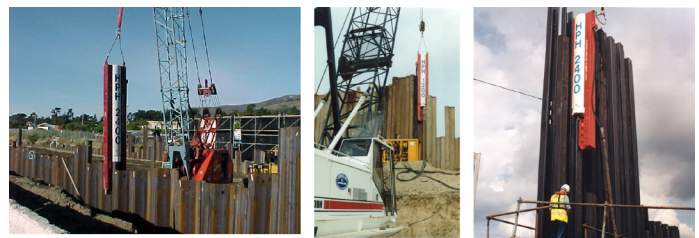
Figure 5-90 Hydraulic Impact Hammer
