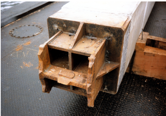
Figure 5-60 H-Pile Points on Concrete Piles
