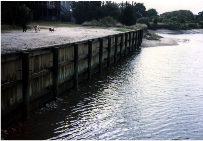
Figure 2-37 Completed Timber Bulkhead
