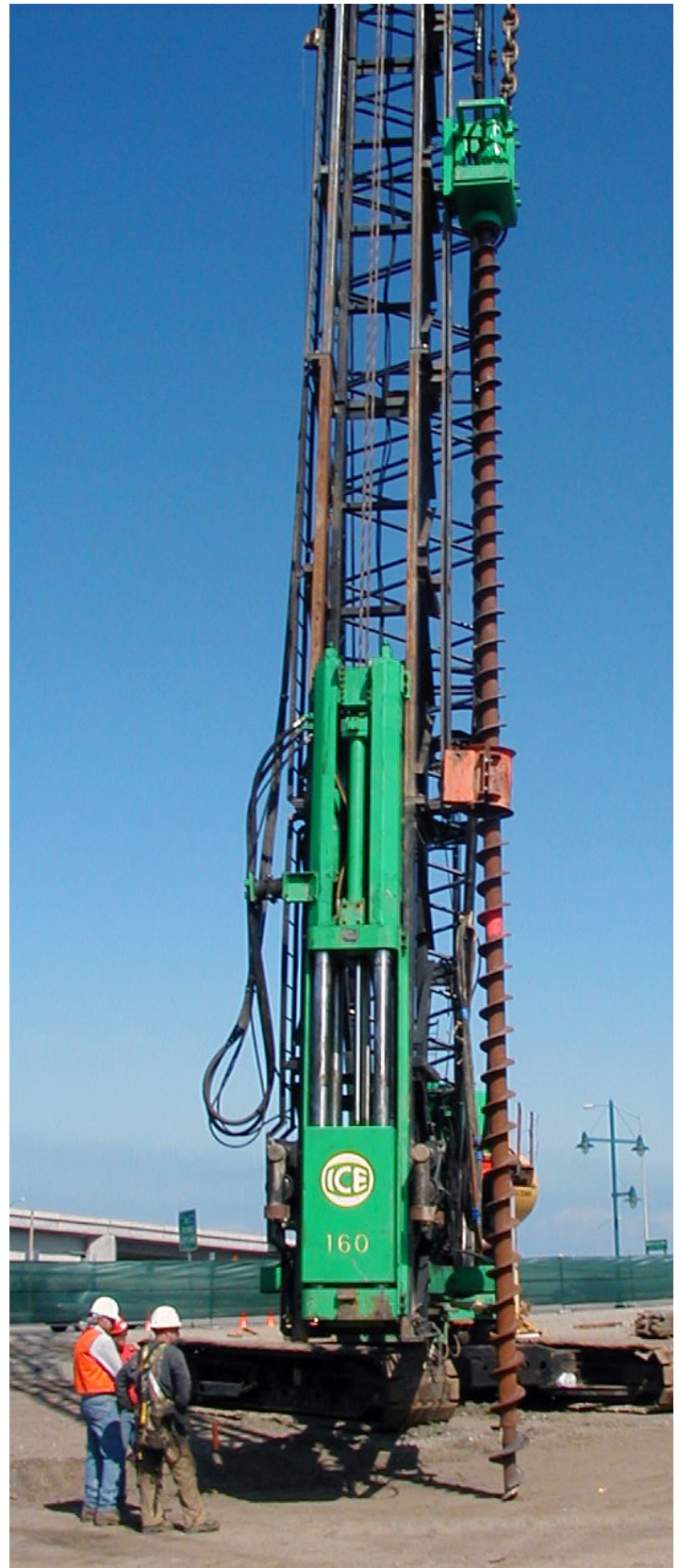
Figure 3-91 Auger Drill with Leaders and Hydraulic Impact Hammer
