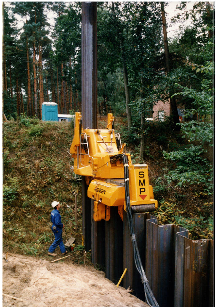
Figure 3-19 Pile Jacking Device for Sheet Piling
