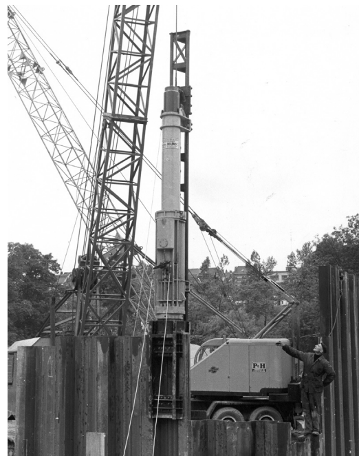
Figure 5-89 Diesel Hammer Driving Sheet Piling
