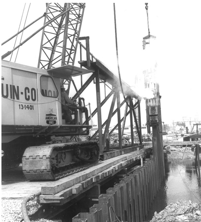
Figure 5-88 Air/Steam Hammer Driving Sheet Piling
