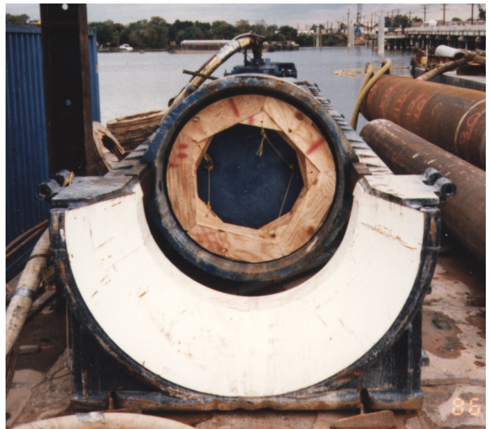
Figure 5-43 Pile Cushion for Concrete Cylinder Pile
