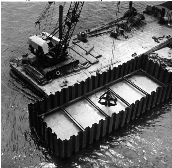
Figure 2-25 Sheet Piling Box Cofferdam
