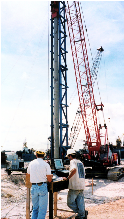
Figure 6-29 PDA Field Test Set-up
