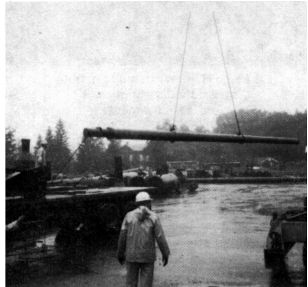
Figure 5-94 Loading Step Taper Core (note tag line to control swing)
