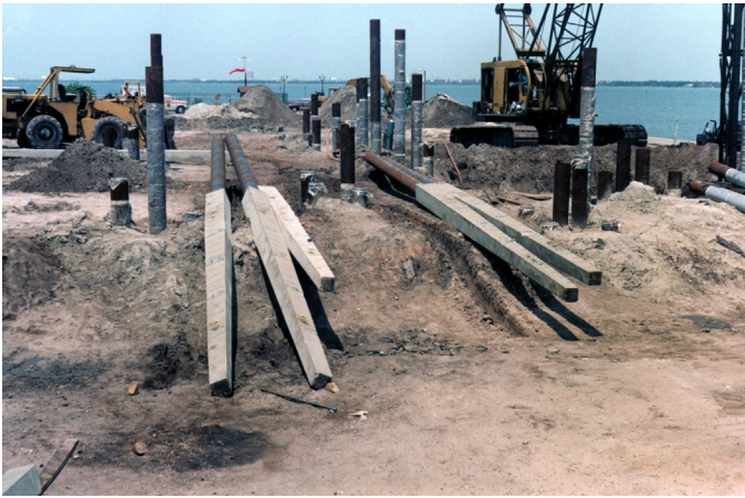
Figure 4-33 Spear Piles for Downdrag Reduction
