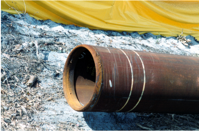
Figure 5-58 Open End Pipe Pile Point
