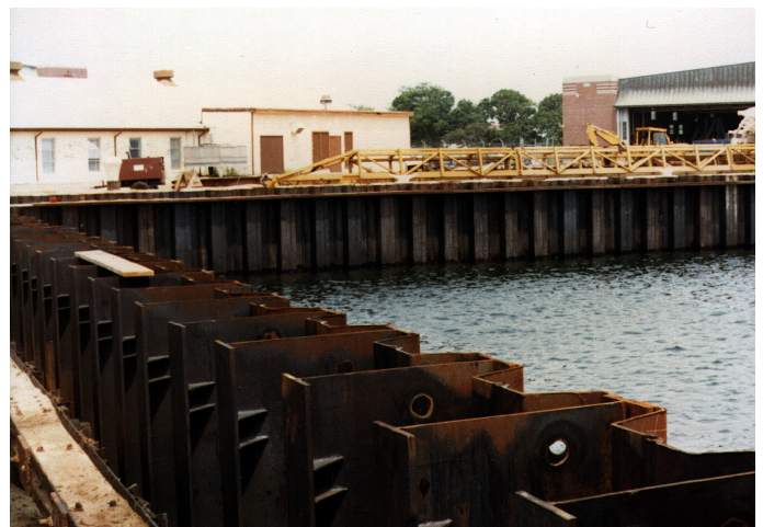
Figure 2-23 Master Pile Wall
