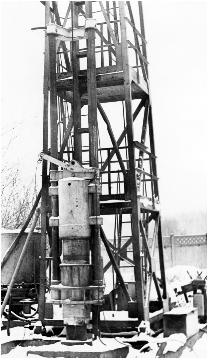
Figure 1-10 Rod Type Diesel Hammer
