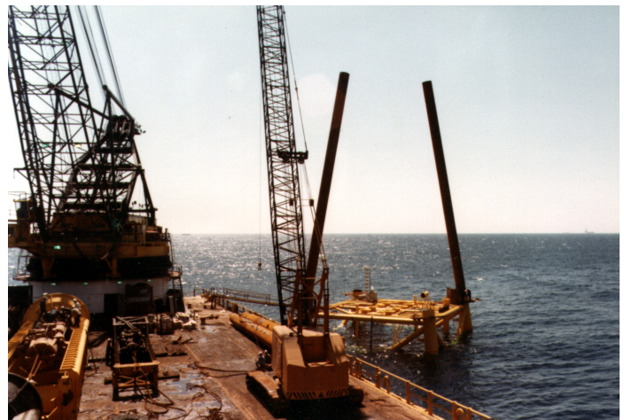
Figure 2-4 Pile Piles for an Offshore Oil Platform
