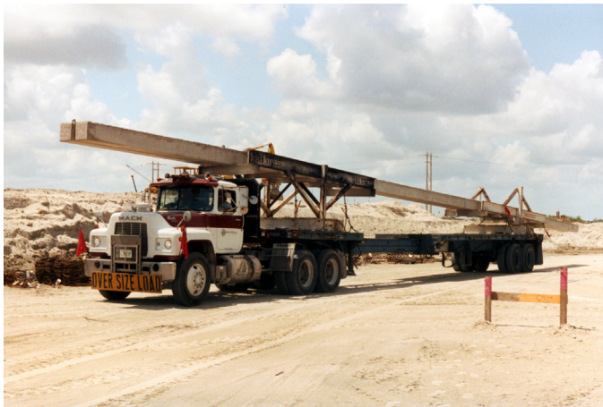
Figure 5-47 Concrete Piles Hauled on Truck
