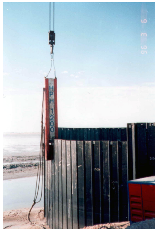
Figure 3-78 Impact Hammer with Pants
