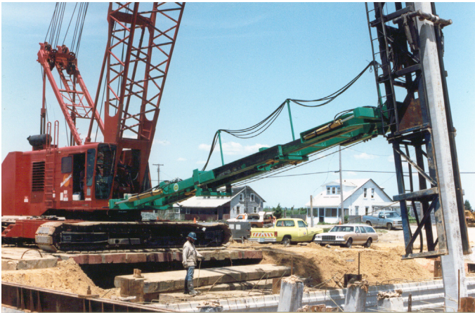
Figure 3-72 Hydraulic Spotter
