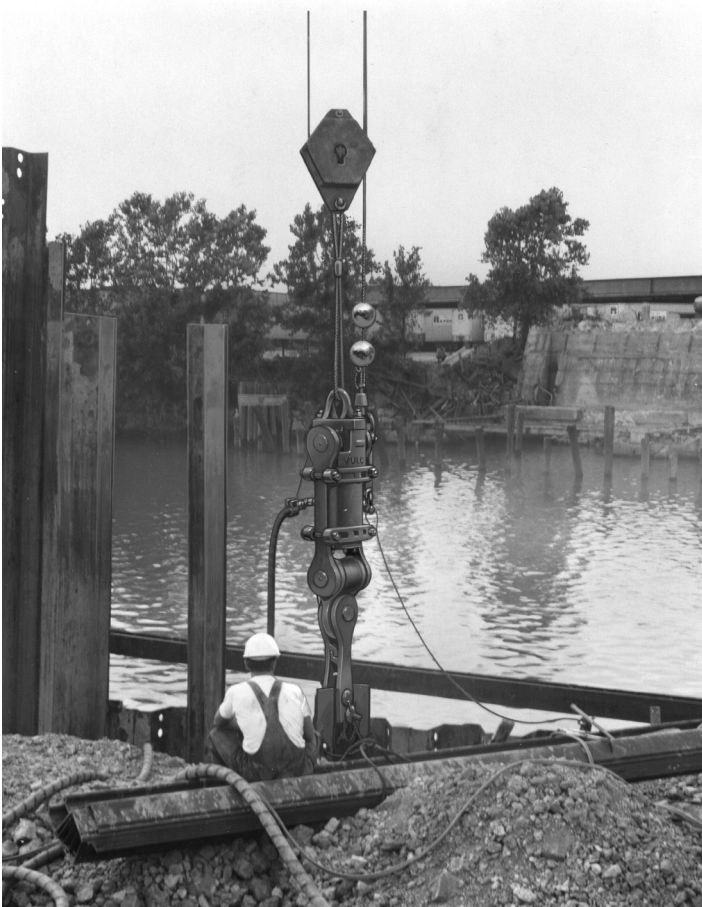
Figure 5-33 Impact Extractor
