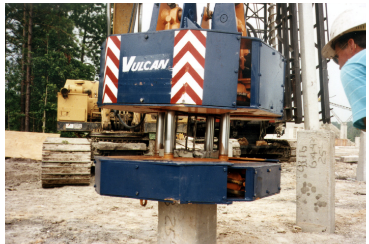
Figure 3-97 Concrete pile cutter
