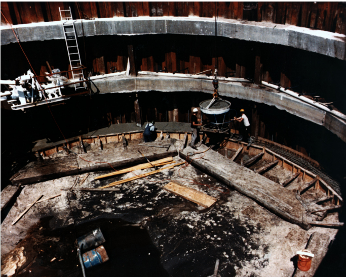
Figure 4-71 Working Inside a Cellular Cofferdam
