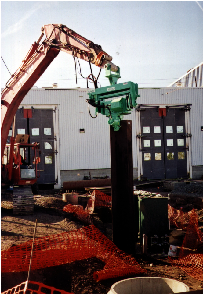
Figure 3-56 Swiveled Excavator Mounted Hammer
