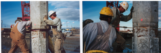
24" oct. Sure-Lock Pile Splice – inserting the top segment Male into bottom segment Female splice half. Driving one of the two locking bars into the grooves of the Male & Female plates with an air hammer to form a circular shear key.
