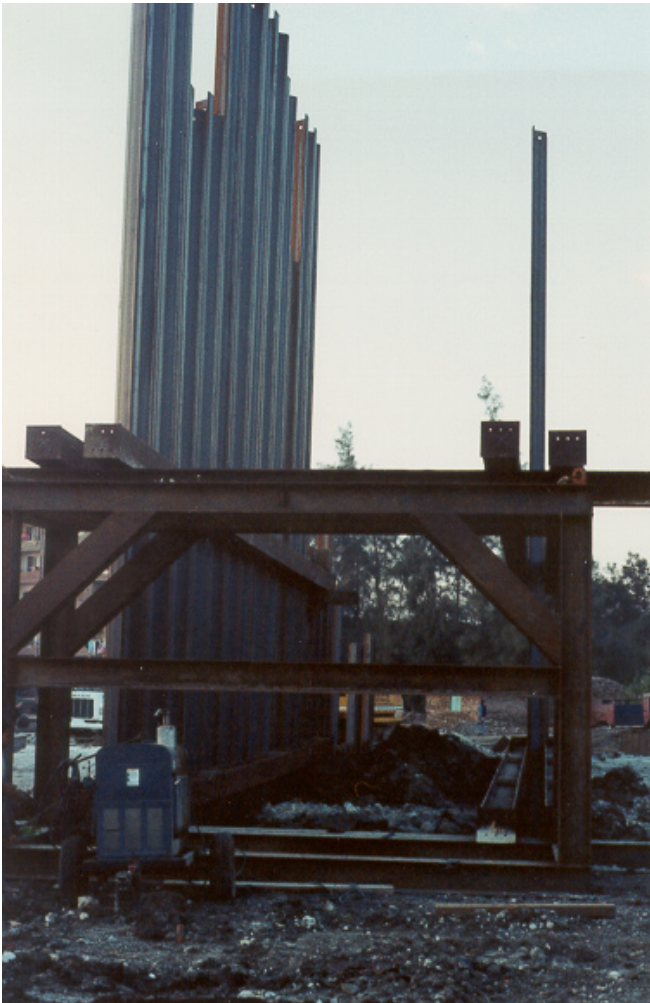
Figure 5-72 Template for Sheet Piles
