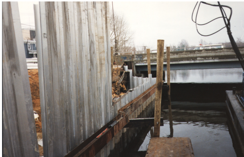
Figure 5-80 Panel Driving in Progress
