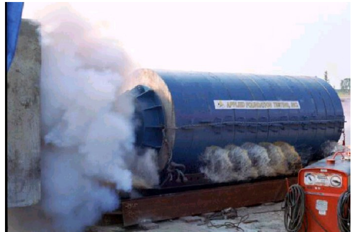
Figure 6-26 Lateral Load Test Using Statnamic™ Device
