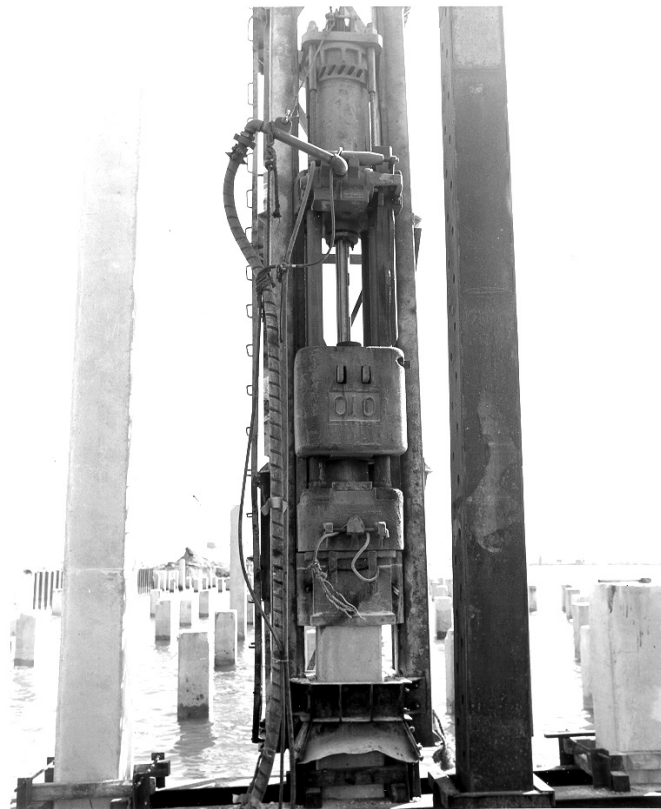
Figure 3-7 Typical Single-Acting Air/Steam Hammer
