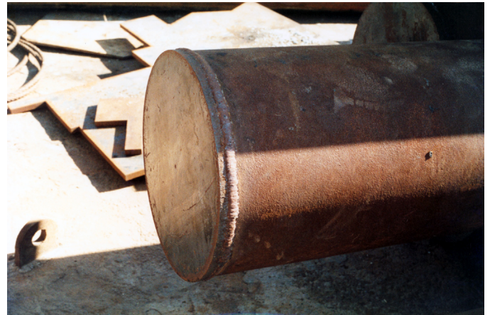
Figure 2-3 Closed End Pipe Piles
