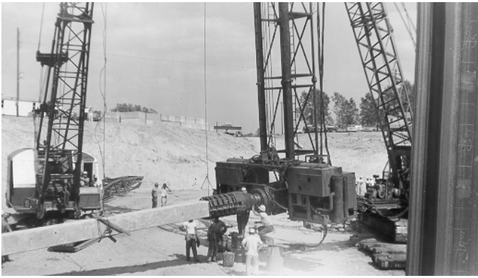
Figure 3-45 Resonant Vibratory Hammer
