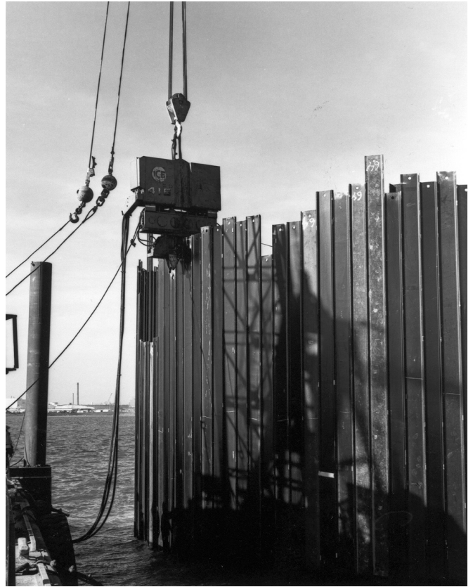
Figure 5-87 Vibratory Hammer Driving Flat Sheeting
