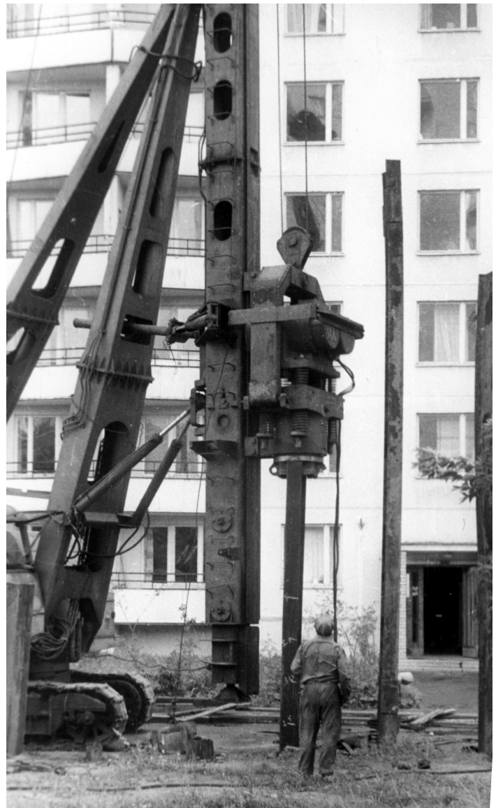
Figure 1-14 Impact-Vibration Hammer
