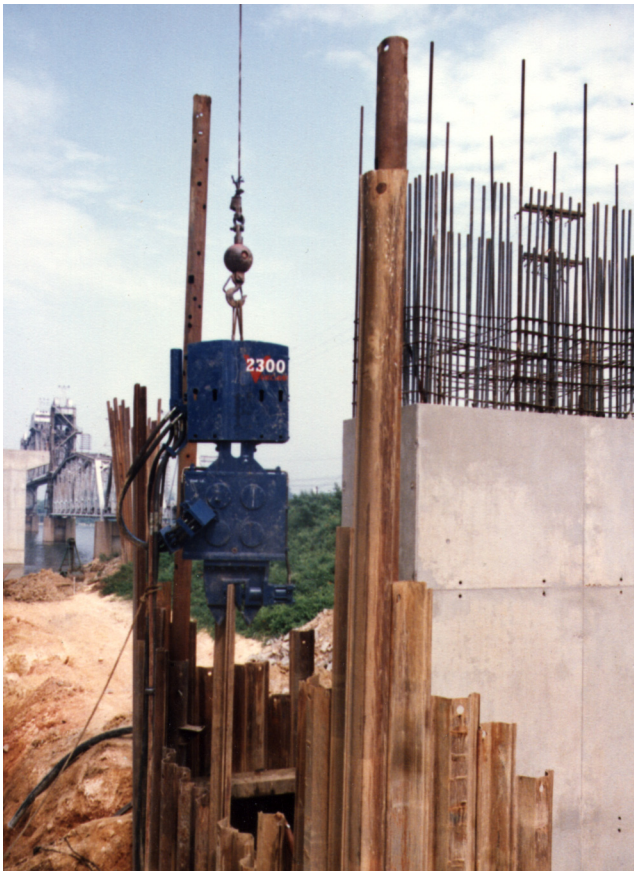
Figure 5-35 Vibratory Hammer Extracting Sheet Piling
