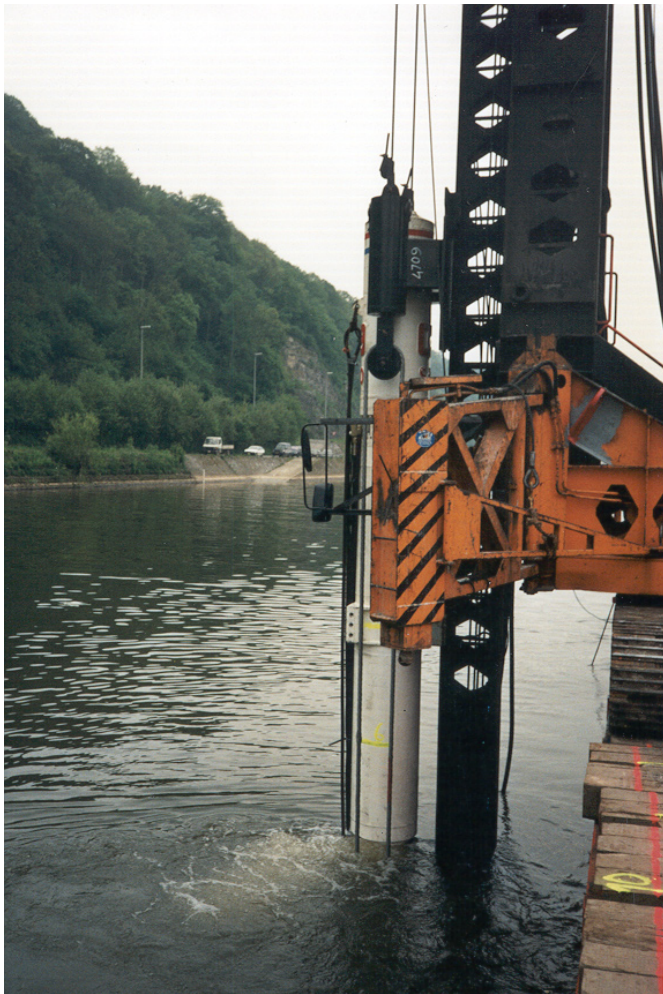
Figure 3-89 Underwater Hydraulic Impact Hammer
