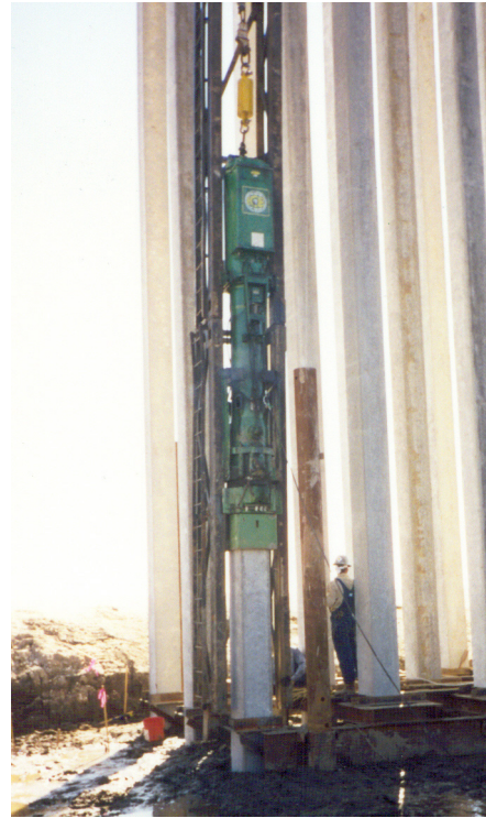
Figure 3-24 Closed End, Double-Acting Diesel Hammer
