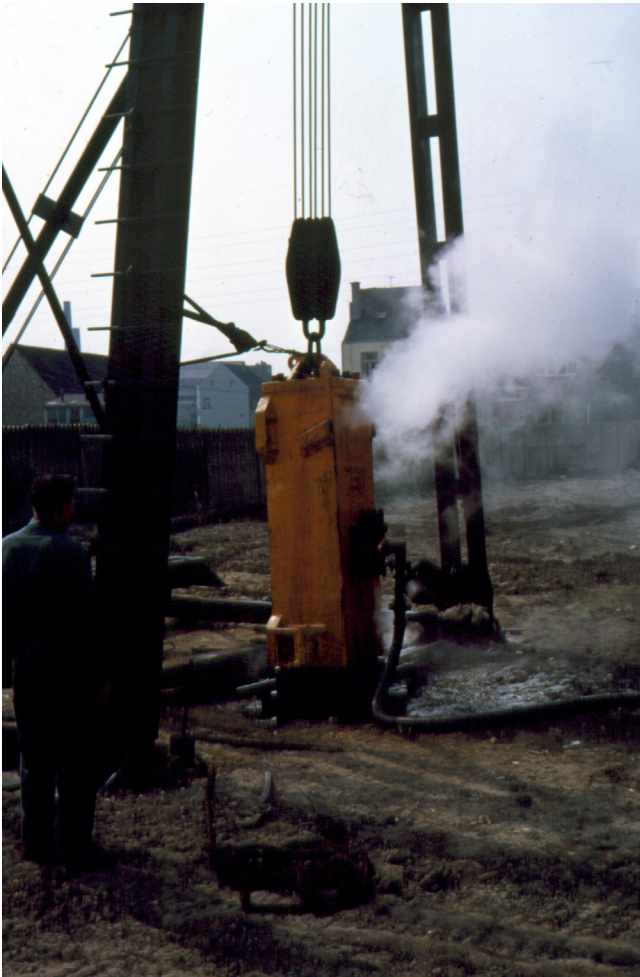
Figure 1-3 Nilens Double-Acting Steam Hammer
