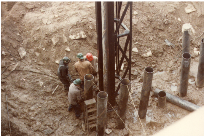
Figure 5-39 Open Head Pipe Piles
