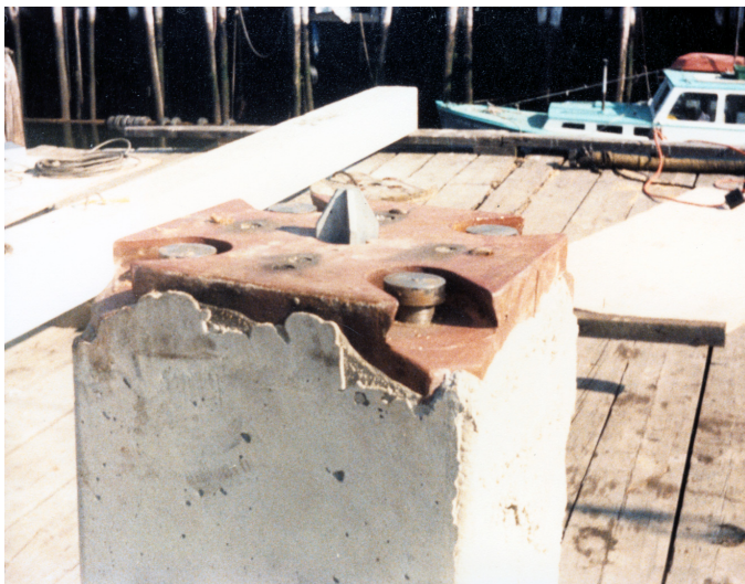
Figure 5-66 Wedge Type Splice
