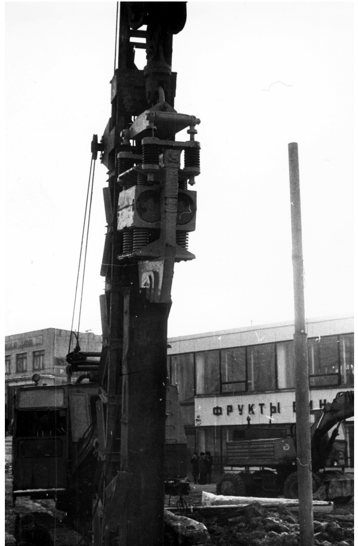
Figure 5-34 Impact-Vibration Extractor
