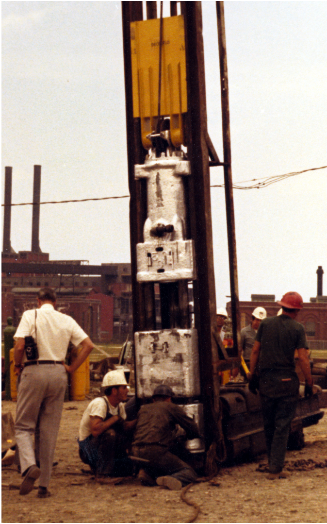
Figure 3-13 Typical Differential-Acting Air/Steam Hammer.
