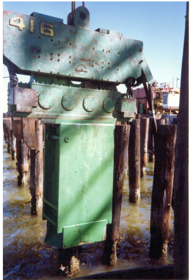
Figure 3-51 Wood Pile Extracted Using Wood Pile Clamp
