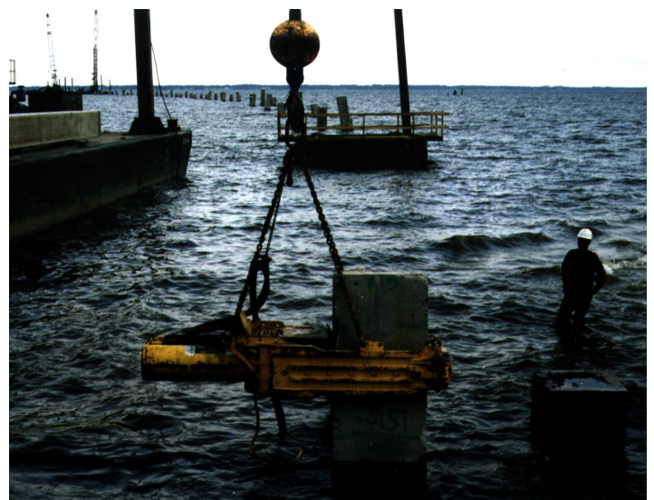
Figure 3-98 Concrete Pile Cutter in a Marine Application
