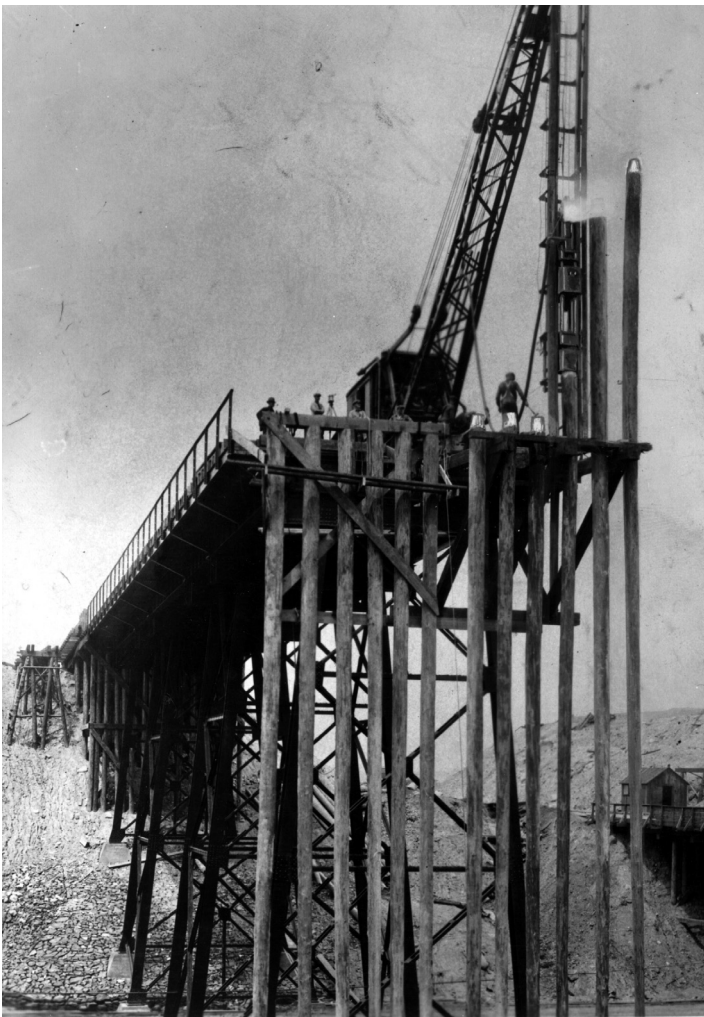
Figure 2-14 Timber Piling Driven for a Bridge
