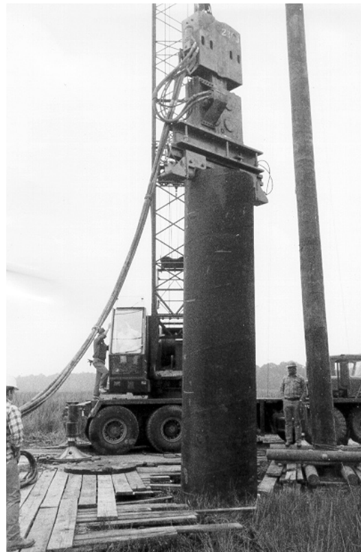
Figure 3-49 Vibratory Hammer Installing Caissons
