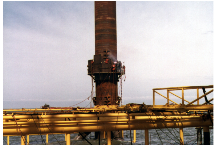
Figure 2-5 Welding an Add-On to Pipe Pile
