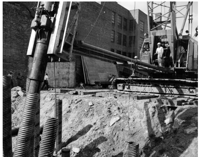
Figure 3-34 Mandrel in Use During Driving
