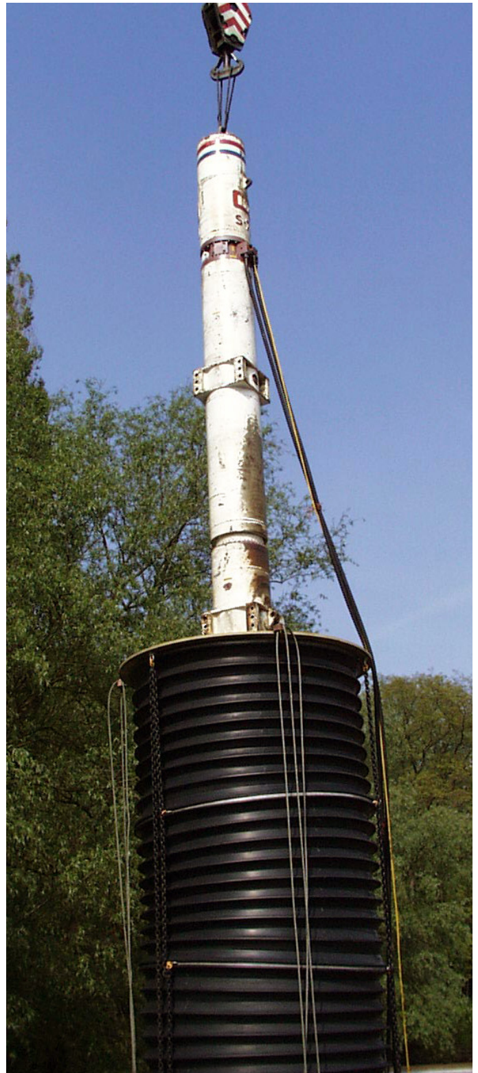
Figure 5-2 Noise Shroud for Pile Driving
