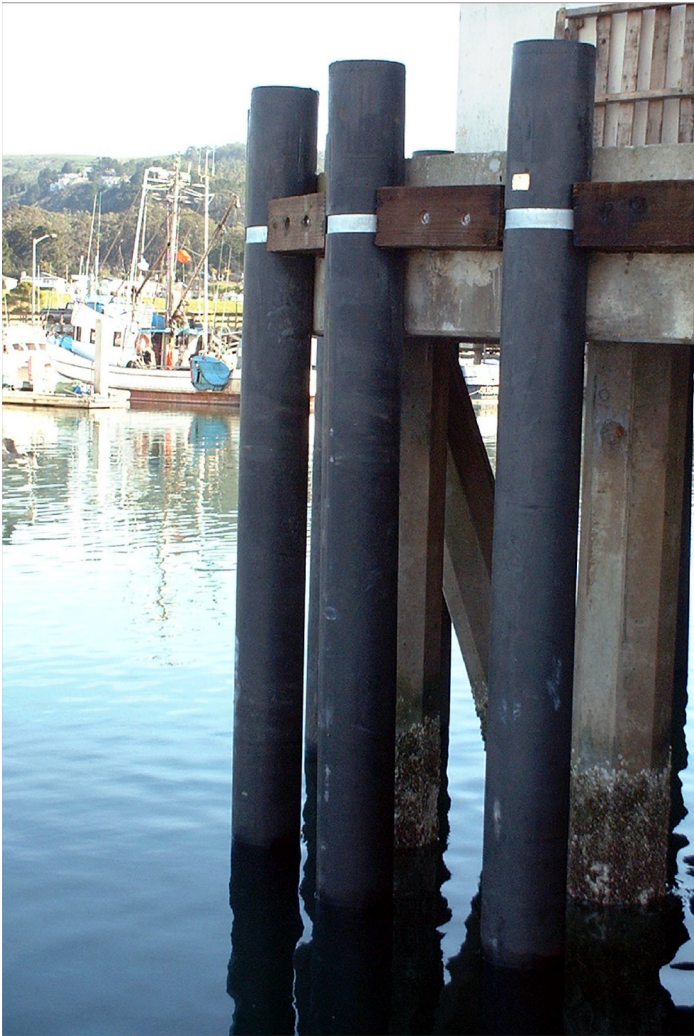
Figure 2-15 Plastic Composite Piling in Marine Application
