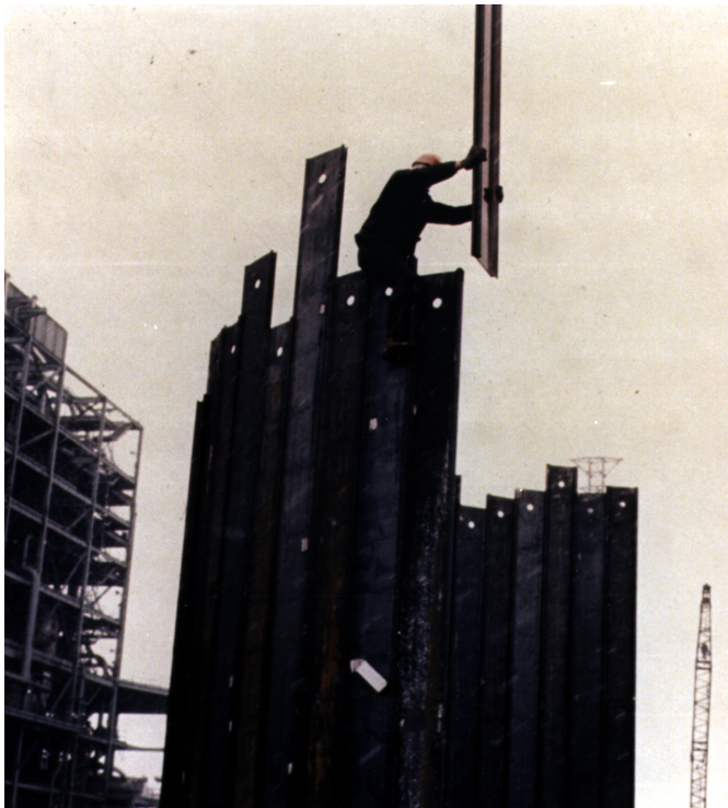
Figure 5-75 Manual Threading of Sheet Piling
