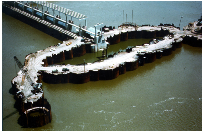
Figure 2-21 Cellular Cofferdam
