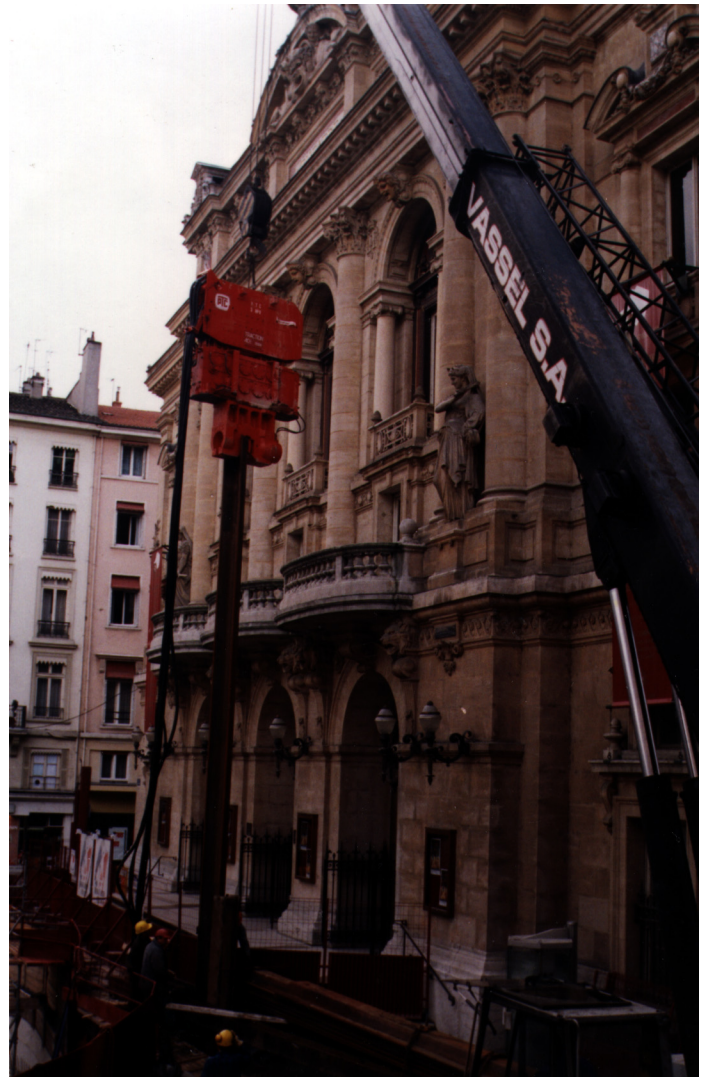
Figure 3-44 High Frequency Vibrator Near Sensitive Structure
