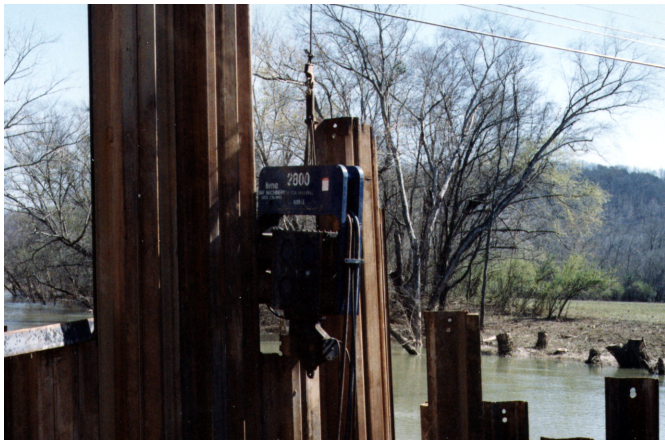
Figure 5-86 Hydraulic Vibratory Hammer Driving Sheet Piling
