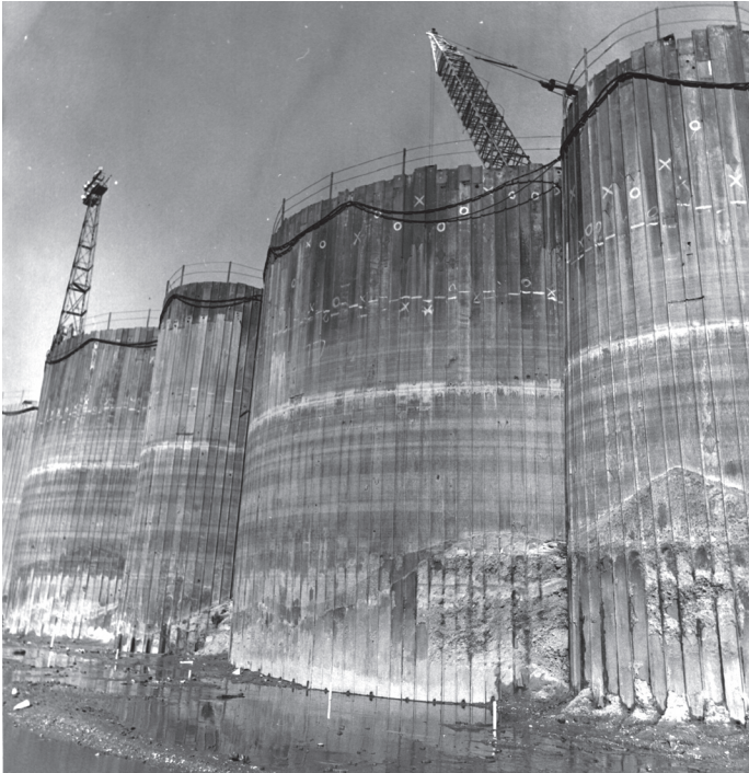
Figure 4-69 Side View of Cellular Cofferdam
