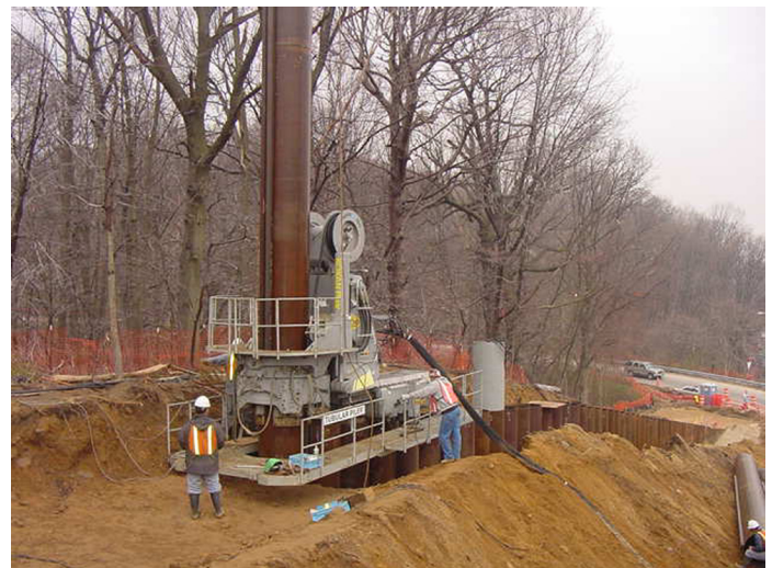
Figure 3-20 Pile Jacking Device for Tubular Piles
