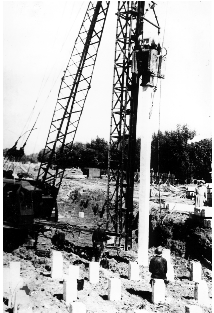
Figure 3-46 Impact-Vibration Hammer
