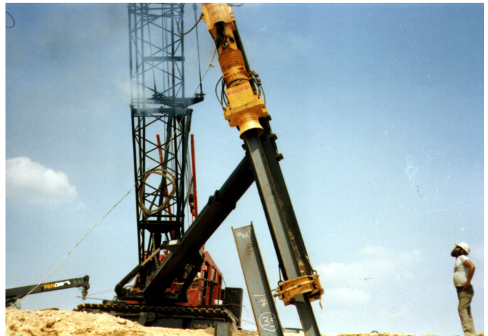
Figure 3-73 Vertical Travel or Semi-Fixed Leaders
