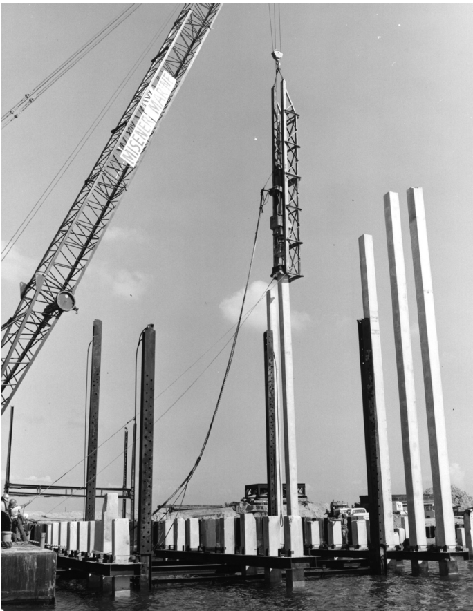
Figure 3-76 Template for Pile Alignment
