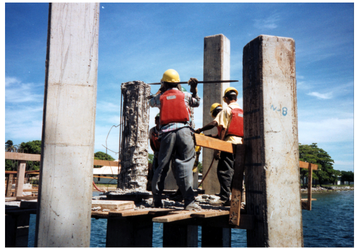
Figure 3-97 Concrete pile cutter
