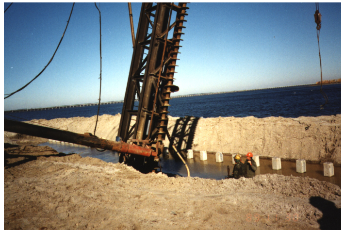
Figure 3-90 Auger Ready to Drill
