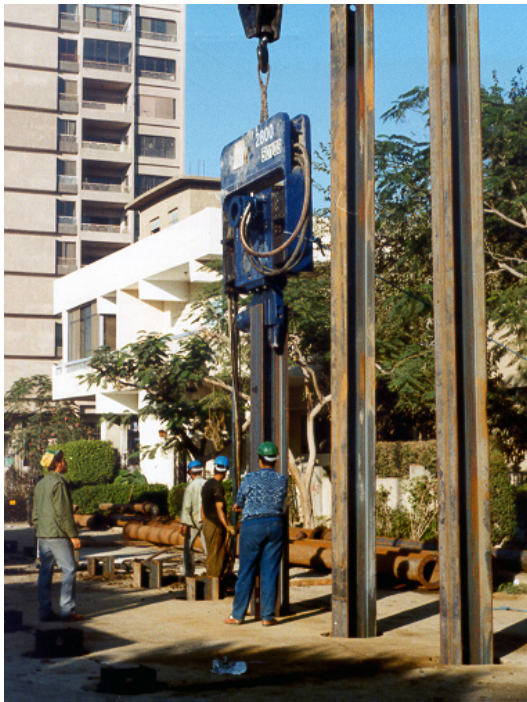
Figure 3-48 Vibratory Hammer Installing H-Piles
