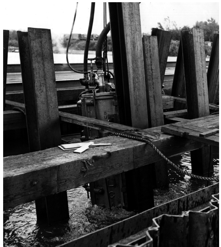
Figure 3-88 Closed Type Differential Hammer Driving Underwater
