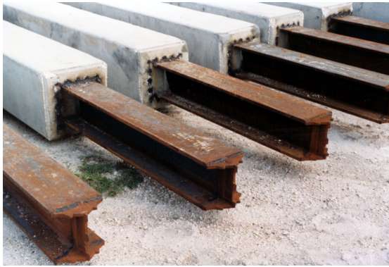
Figure 2-10 H-pile “Stinger” on Concrete Pile
