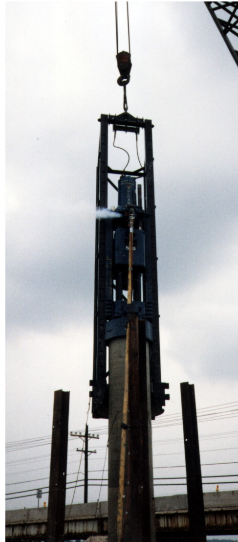
Figure 5-49 Driving 54" (1371.6 mm) Pile
