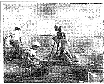
Individual Flexifloats are quickly and rigidly secured together.
